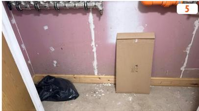
General housekeeping issues were noted throughout the means of escape, i.e. boxes/ combustibles/general obstructions etc. Remove the obstructions and maintain the means of escape clear.
